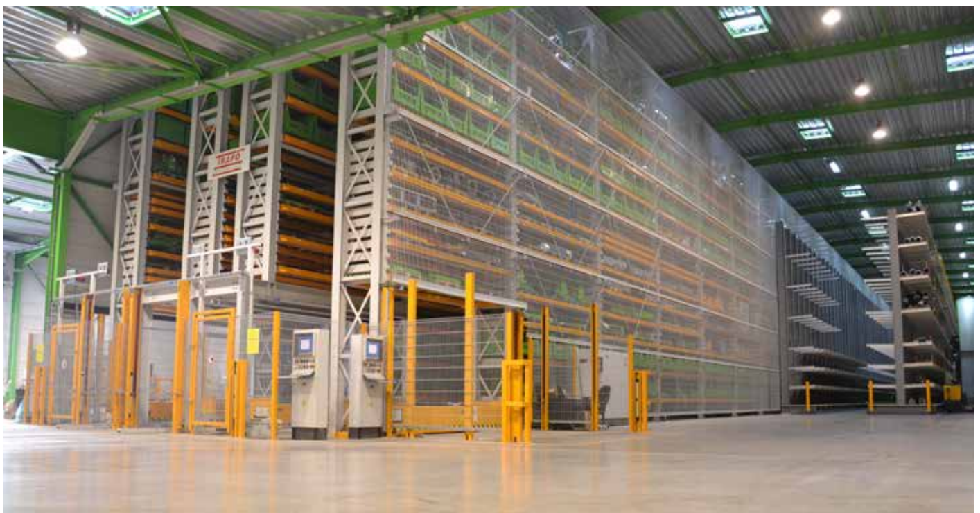
Automated Storage Area of 28.000m 3
